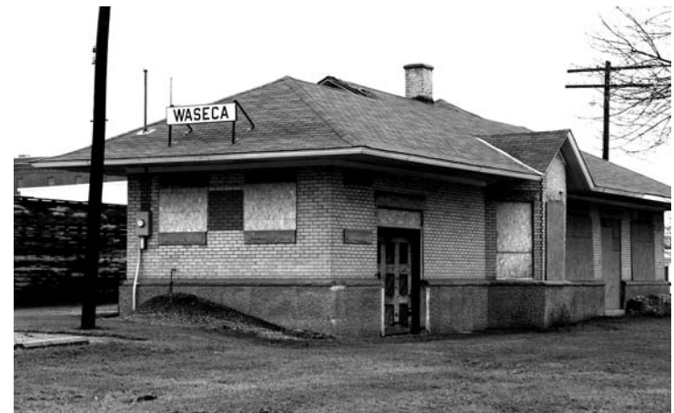
A renewed effort is needed to save the Waseca passenger depot, one of the Alliance's 10 Most Endangered properties in 2007
